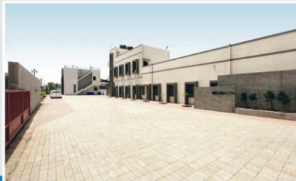
Our State of Art New Mfg. Facility
